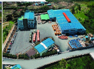
3rd Factory (히트펌프 전장판넬)
