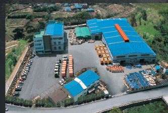
3rd Factory (히트펌프 전장판넬)
